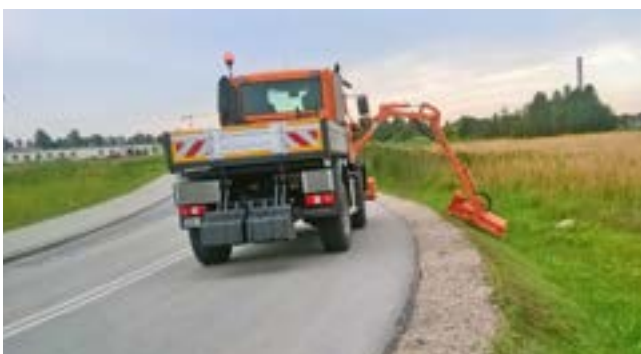
Mowing of a hard-to-reach roadside using a WWP500UH multifunction arm and GK 110 head
