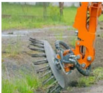
Removing vegetation from around curbs
